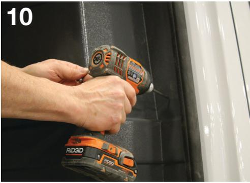
Loosely secure the sides with 3/4" self-tapping screws (E).
